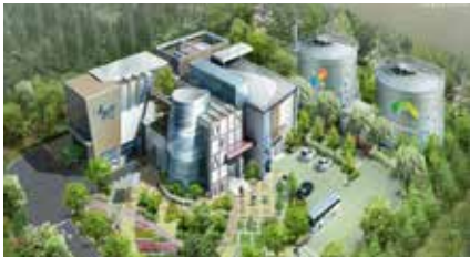
오폐수처리장 WASTEWATER TREATMENT PLANT
